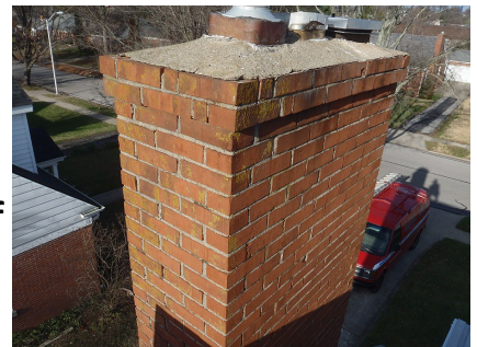
Photo of entire chimney from roof
