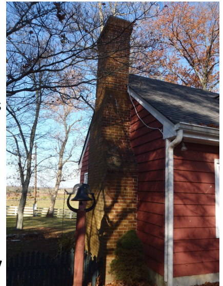
Photo of outside of chimney
